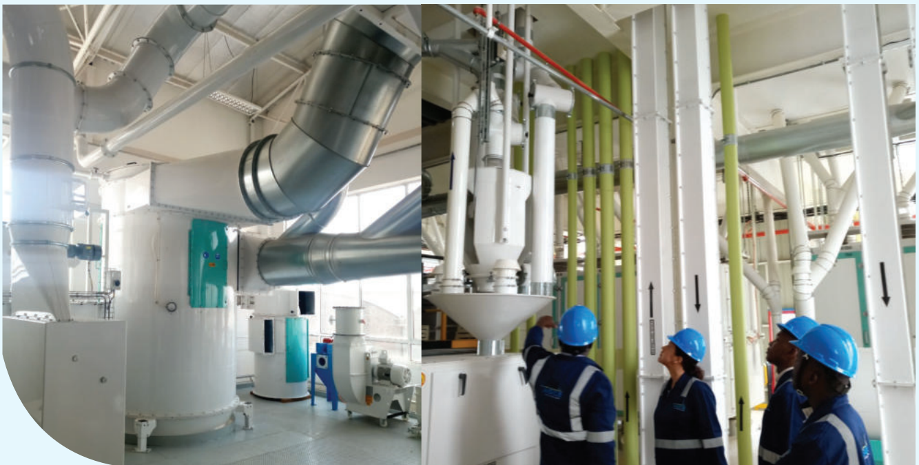
Eldoret Unga Ltd Mill Installation
