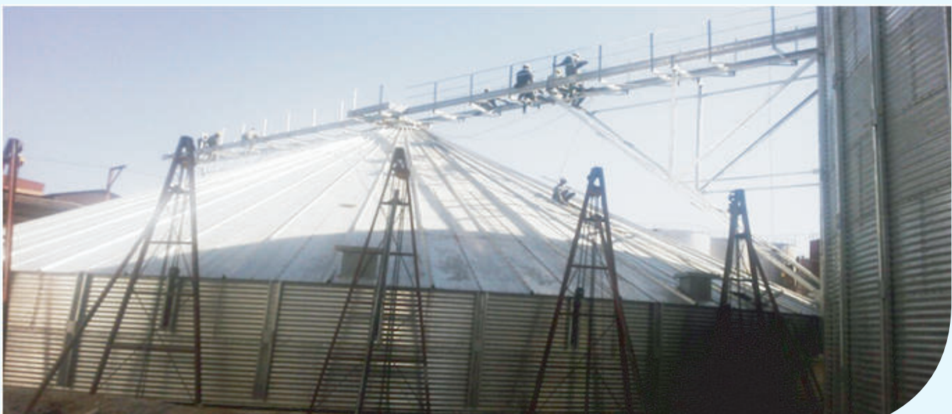
Mt. Meru Millers, Singida Tanzania, Silo Installation 2016
