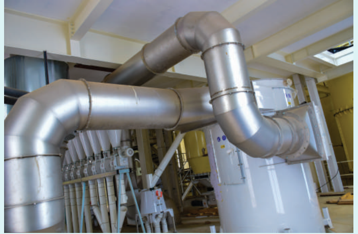
Dust Filter, Aspiration Pipes and Air Locks
