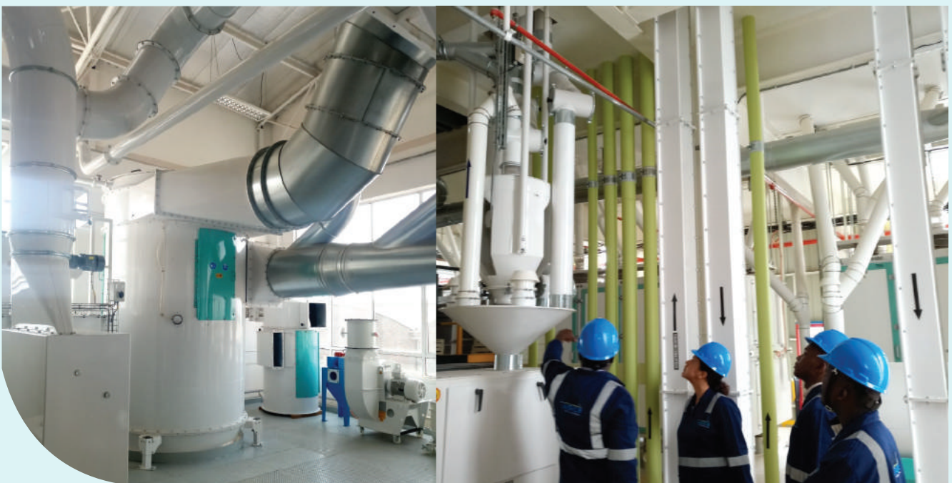
Eldoret Unga Ltd Mill Installation
