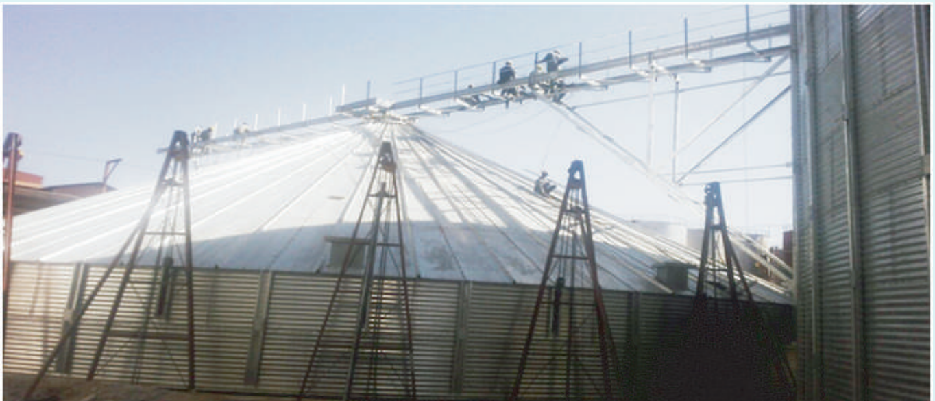
Mt. Meru Millers, Singida Tanzania, Silo Installation 2016
